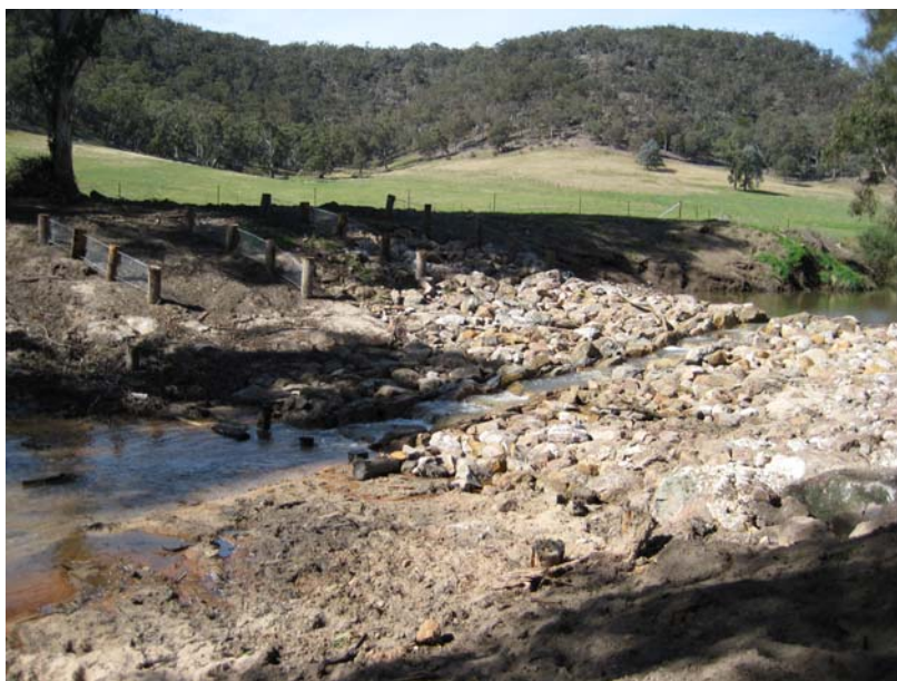
Figure 6.4: Black Bobs Creek fishway and bank stabilisation works
